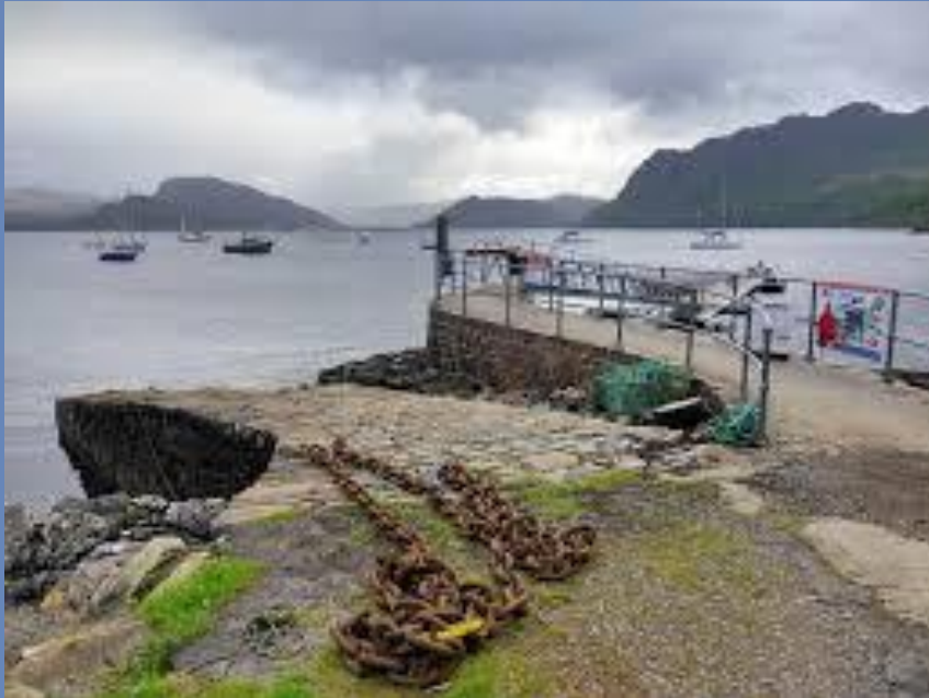
PLOCKTON MAIN PIER PONTON
